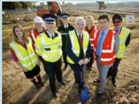
David Jamieson at the start of building work of the new custody block in Perry Barr
